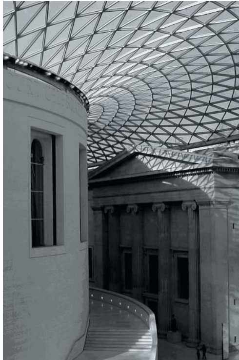
Figure 1. The Great Court Roof.
